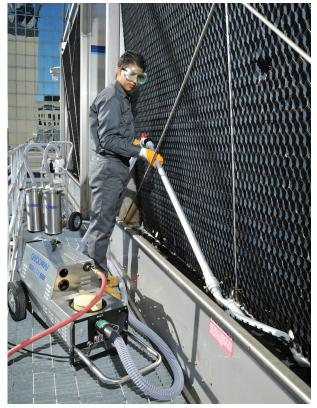
**ONLINE CLEANING:** Clean and filter your cooling tower water without having to drain the system or shut it down.
