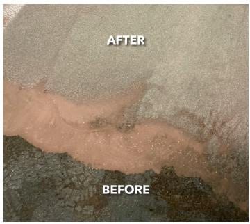
The dry steam and floor spinner combination quickly cut through the buildup, getting the debris removed entirely from the surface.
