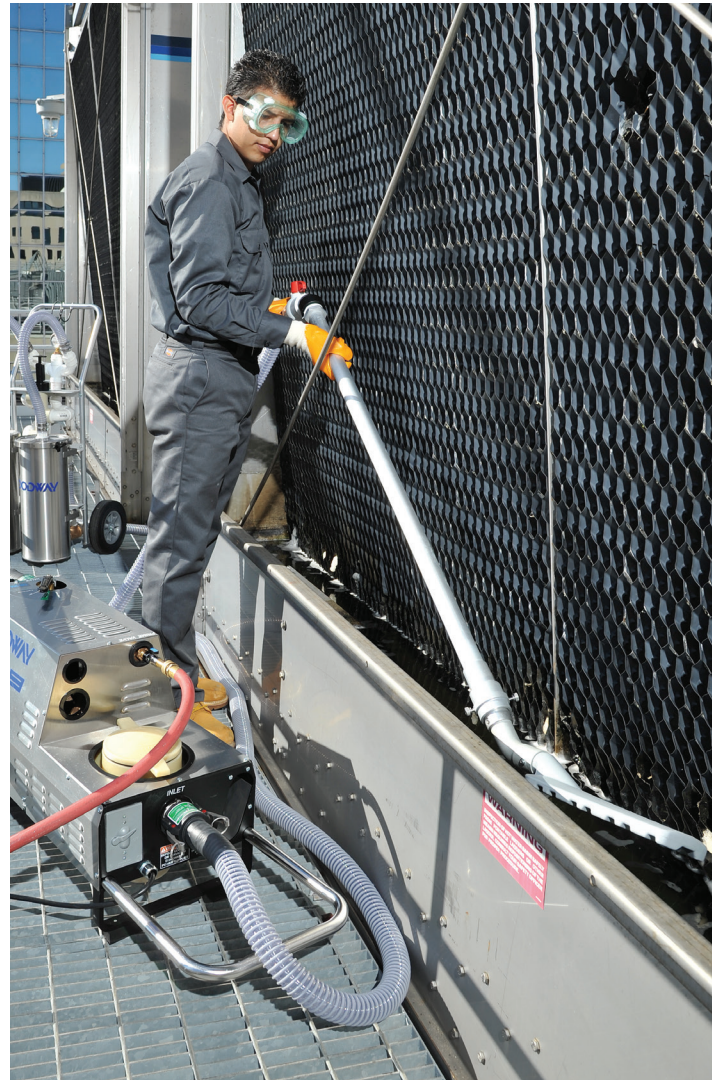
Online Cleaning: Clean and filter your cooling tower water without having to drain the system or shut it down.
