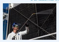
Goodway's ScaleBreak-Gel is a patented, innovative viscous gel formulated for descaling vertical surfaces like cooling tower fill. When used in conjunction with Goodway's TFC-200 system, ScaleBreak-Gel adheres to vertical surfaces allowing its powerful descaling properties to penetrate and dissolve water formed deposits into a liquid suspension for easy removal.
