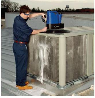
>CLEAN FROM THE INSIDE OUT: Clean against the airflow to flush dirt back out the way it came in.
