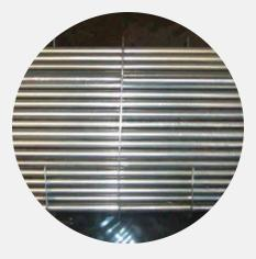
Scale accumulation can lead to energy inefficiency. Scale can act like an insulation barrier on the heat transfer surface, which can result in poor heat transfer. In this situation, a corresponding increase in energy usage is required to achieve the same output.
