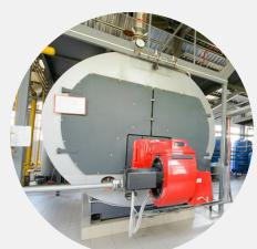
According to the EPA, a fire tube boiler using 450,000 MMBtu of fuel (at \$8.00 per MMBtu) over 8,000 hours per year with 1/32 inch of normal scale translates to a yearly operating cost spike of more than \$70,000.
